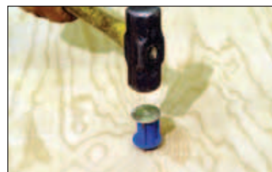
Wood-Form Insert Installation Sequence
