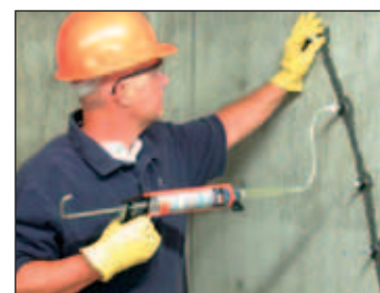
Crack-Pac® injection epoxy using the E-Z-Click Port System
