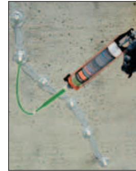
For Leaking Cracks
