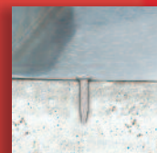
Perimeter Steel to Concrete #55134
