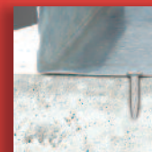
Steel to Concrete #55132
