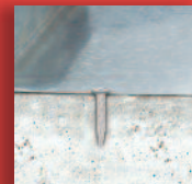
Perimeter Steel to Concrete
