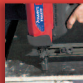
Plywood to Concrete
